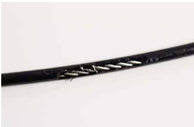
A TEAR IN THE CABLE COVER
