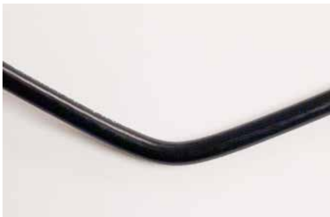
A BREAK ON THE CABLE
