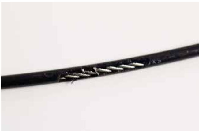
A TEAR IN THE CABLE COVER
