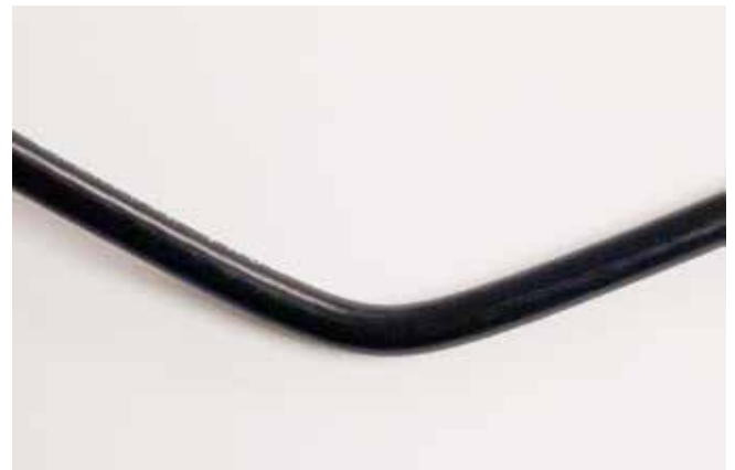
A BREAK ON THE CABLE
